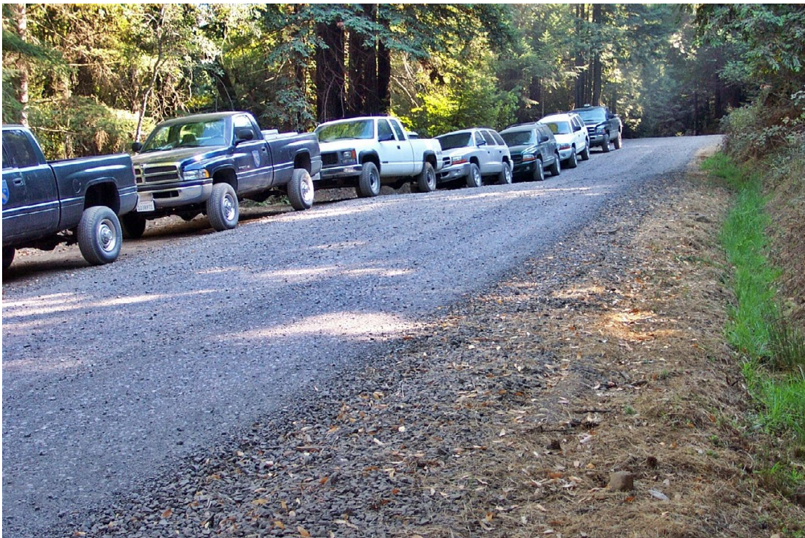
FIGURE 43. This rural subdivision road has been converted from an insloped, ditched road to an outsloped road shape with rolling dips and an inside ditch. Broad rolling dips have been built at regular intervals to accommodate all traffic types. The ditch has been retained to drain clear spring flow from the small cutbank. The road surface no longer drains to the ditch.
