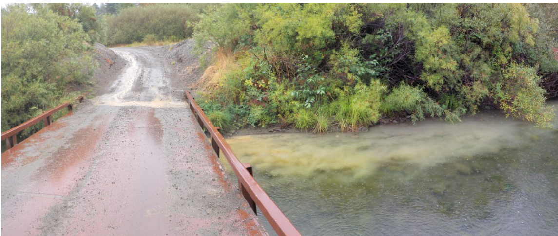
FIGURE 21. Road approaches to bridges are often hydrologically connected. This through cut approach to a temporary bridge drains directly into the stream.
