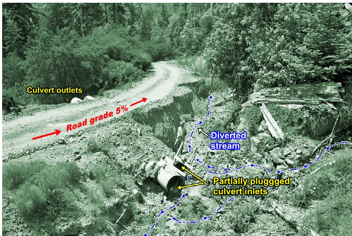
FIGURE 66A. Double culvert stream crossing showing the result of a stream diversion that occurred during a winter storm. The road slopes to the distance at about 5 percent. When the culverts plugged with debris, streamflow diverted down the inboard ditch and created the large diversion gully. Note the person for scale.
