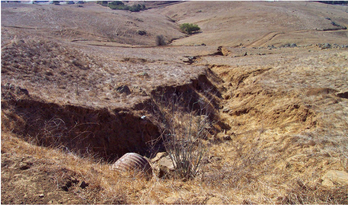
FIGURE 45. If ditches show excessive erosion, or long gullies form below the outlet of a ditch relief culvert, then the ditch is carrying too much flow and additional ditch relief culverts are needed up the road to break up the flow. Gullies below culvert outlets are a common source of hydrologic connectivity, delivering road runoff and eroded sediment to the downslope stream channel.
