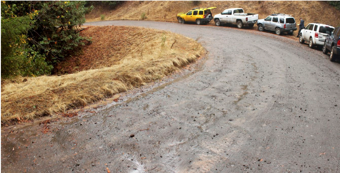
FIGURE 82. This newly upgraded stream crossing fill was protected from road runoff and erosion by the installation of a drainage berm along the road. Once the fill is vegetated and stabilized, the berm can be safely removed.
