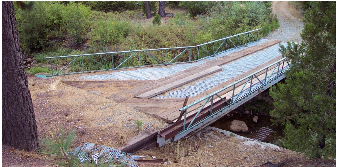
FIGURE 118A. This railroad flat-car bridge has been structurally modified to allow for some truck turning on the bridge deck. Deeply incised stream channels with steep sideslopes would require extensive hillslope excavation if a straight approach was utilized.
