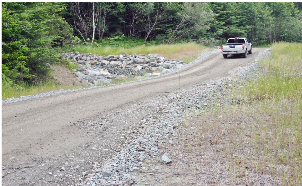
FIGURE 69. A gradually climbing road changes grade over the small stream crossing, thereby eliminating the possibility for future stream diversion. The dip is broad and gentle to accommodate all traffic, and designed to carry peak flood flows across the road and back into the channel with minimal erosion and sediment delivery.
