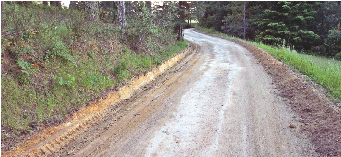
FIGURE 41. This outside berm on a crowned road prevents road surface runoff from draining onto the adjacent hillslope. If the road was insloped, the berm would not interfere with road drainage.
