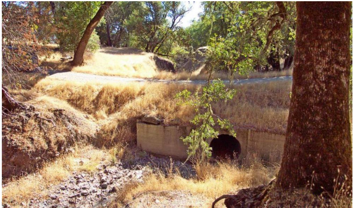
FIGURE 111. This concrete vertical headwall was installed on a ranch road stream crossing. The headwall increases culvert efficiency compared to a projecting barrel inlet, but is still prone to plugging by floating organic debris.
