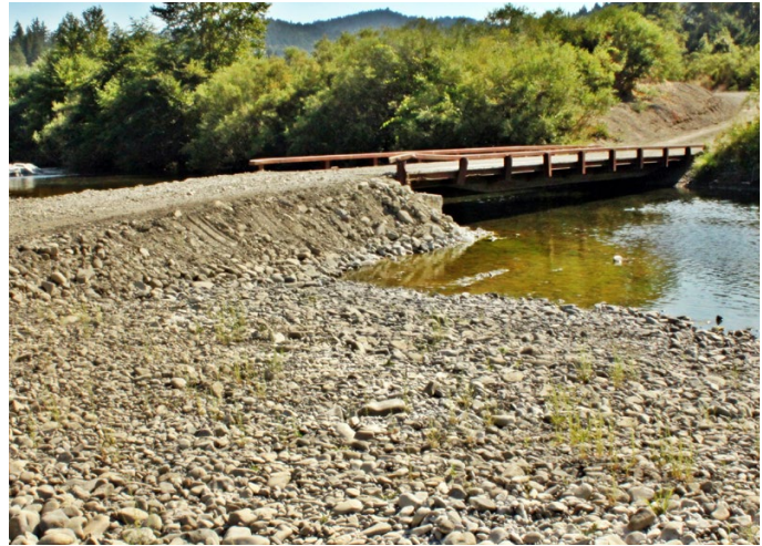
FIGURE 127B. A temporary bridge crossing should be used where migrating adult or juvenile fish need to pass beneath the crossing. This temporary bridge crossing spans the active summer channel and the abutment in the channel is composed entirely of clean stream gravels. All temporary low water crossings should be removed before the first seasonal rains.
