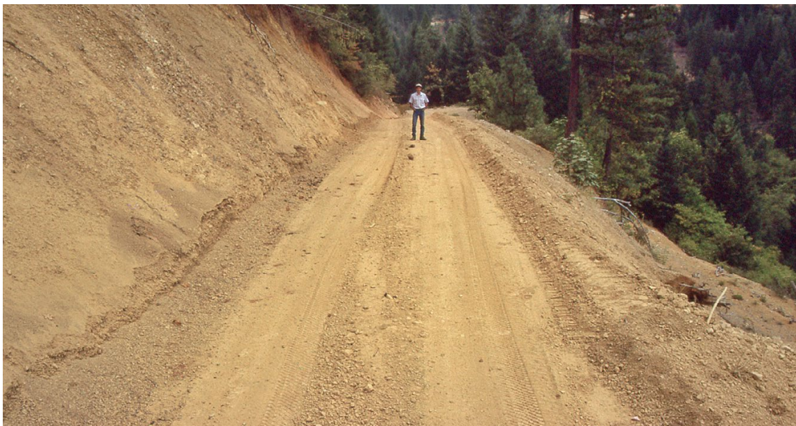
FIGURE 42. Short road reach where a soil berm has been intentionally constructed along the outside edge of the road prism to prevent surface runoff from flowing over the highly erodible fill. To prevent the accumulation of too much runoff, the berm can be intermittently breached and a small flared inlet and culvert or sheet metal berm-drain installed to carry runoff downslope past the base of the erodible fill slope.
