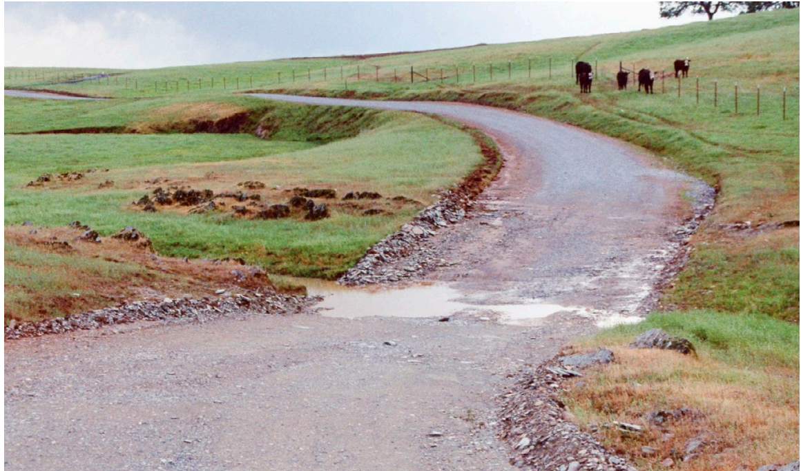
FIGURE 125. In addition to the actual ford crossing, the road approaches also contribute to sediment pollution unless they are paved or heavily rock surfaced. Fords are always low points in the road, so runoff from the connected approaches is delivered directly to the stream channel.
