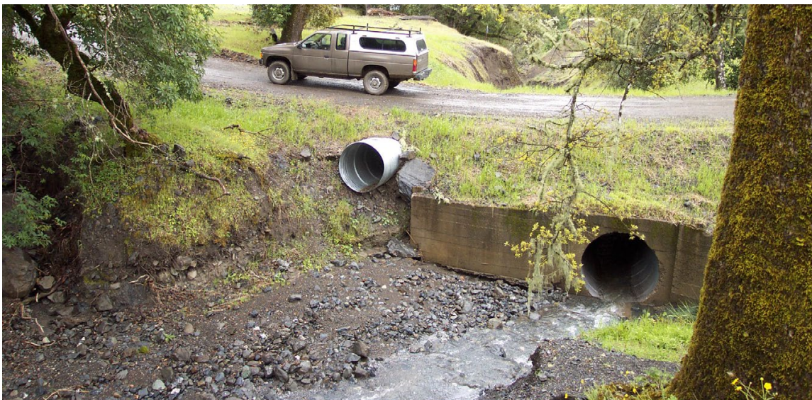
FIGURE 115. Where stream crossing culverts may not be adequately sized for the design flood flow, and they are not scheduled for immediate replacement, they can be fitted with more efficient entrances (such as the headwall seen here) as well as emergency overflow pipes installed higher in the fill. The overflow pipe provides relief during the large flow events or when the main culvert becomes plugged with debris. This overflow culvert experienced flood flow during the first winter after it was installed (See Figure 111).
