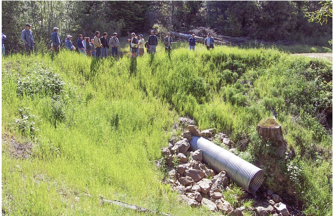
FIGURE 80. Rock armor placed around this culvert where it emerges from the fill slope was used to protect the stream from unexpected erosion of the new, erodible fill slope until it stabilized with vegetation.
