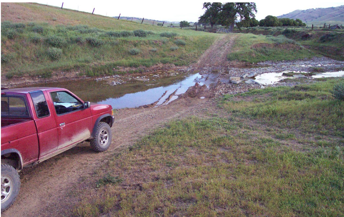
FIGURE 124. This unimproved ford crossing of an intermittent stream was poorly located in a channel reach that had a fine, erodible bed. Efforts to stabilize the channel bottom with rock and concrete chunks have been unsuccessful. A plume of turbidity is released in this fish bearing channel with each crossing.
