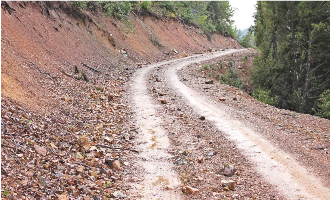
FIGURE 23. Full bench road. The height of the cut-bank, the slope of the natural hillside and the small amount of sidecast indicates that this road is full bench and cut entirely into native hillslope materials. Note that the road has no inboard ditch.
