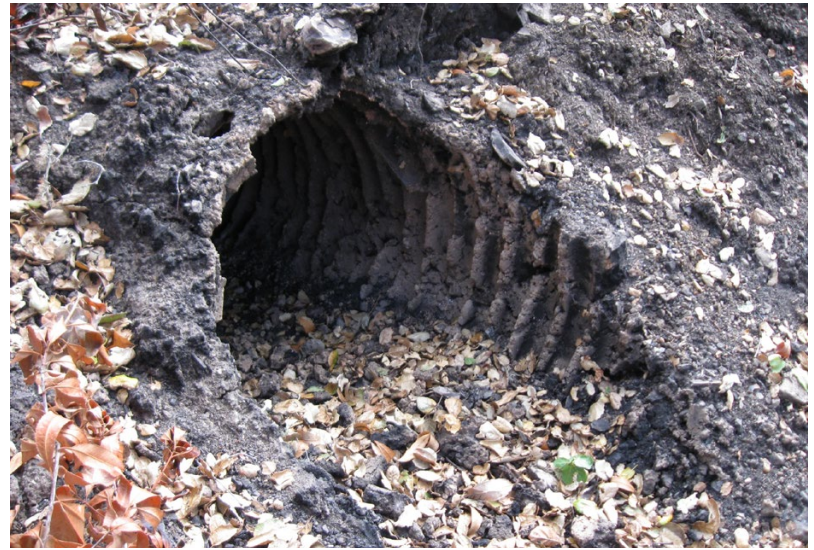
FIGURE 87. This plastic culvert was melted and burned out during a forest fire in central California. In fire-prone areas, metal culverts may be more suitable, or plastic culverts can be fitted with metal inlets and outlets that prevent burning (Pete Cafferata, Calfire).
