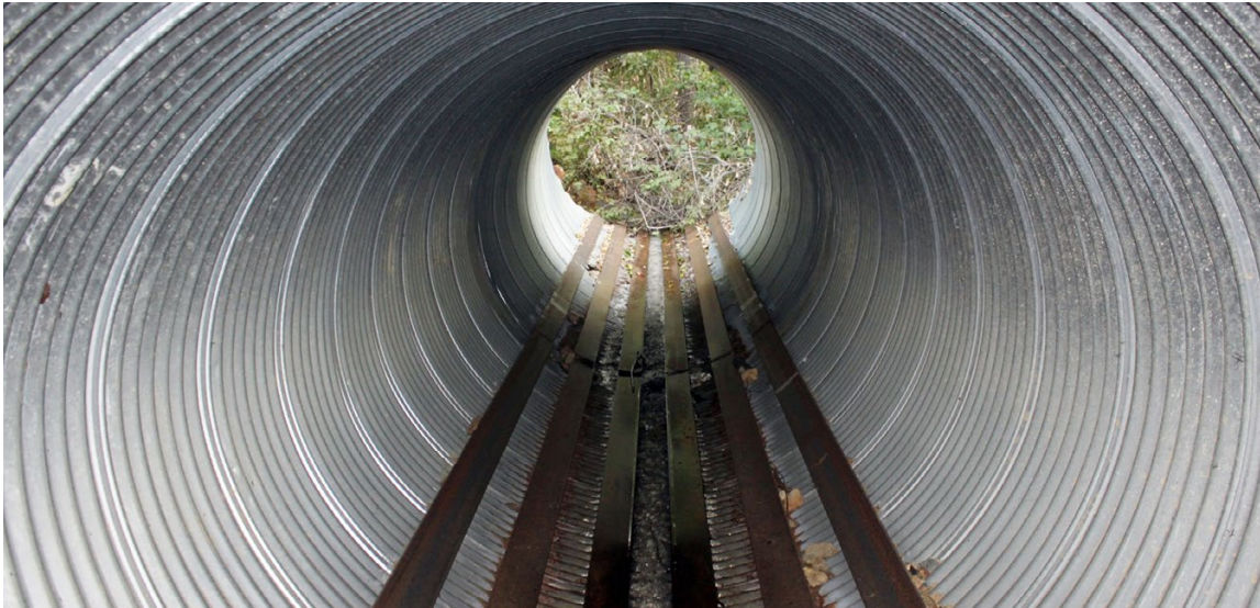
FIGURE 89. Steel plates have been welded onto the lower 25% of the invert of this 6 ft diameter galvanized culvert. The steel provides protection against abrasion by coarse bedload transport.
