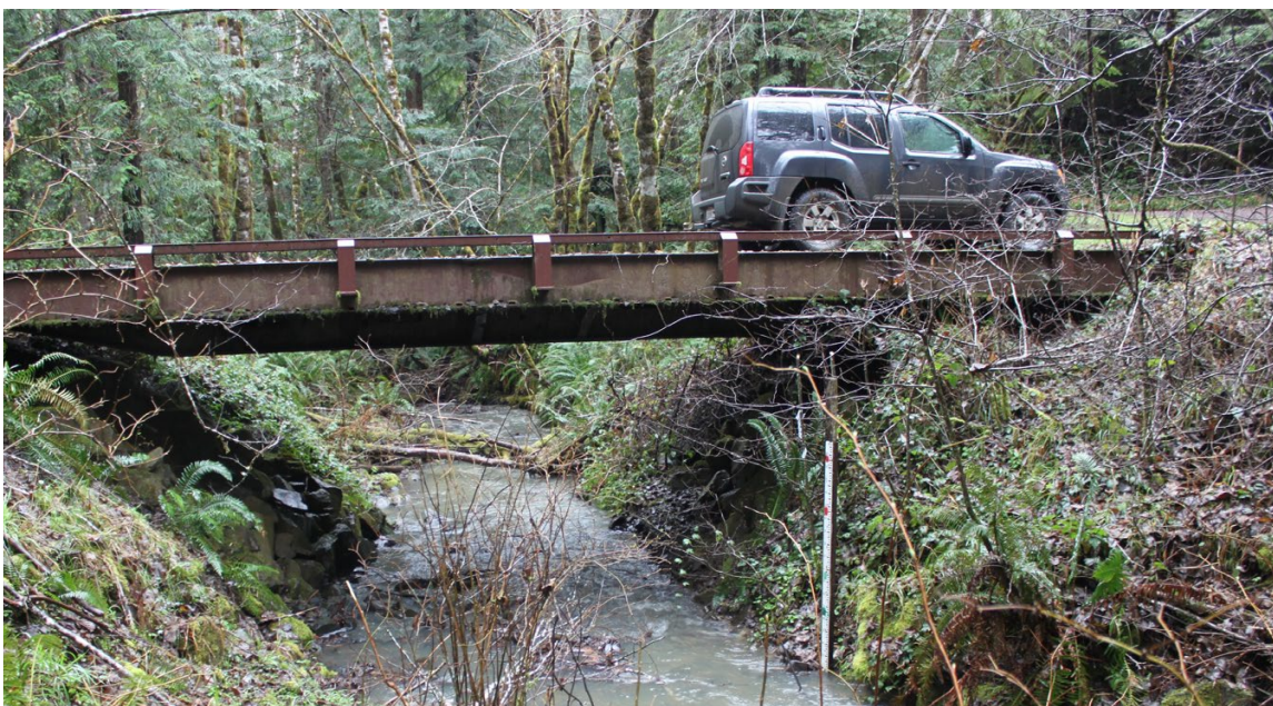
FIGURE 71. This 45-foot railroad flatcar bridge was installed to replace an undersized culvert that had been a barrier to fish migration. The channel width was maintained and a minor amount of armor was used to protect the abutments from erosion.
