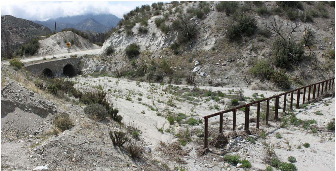
FIGURE 105. In larger streams, debris racks may need to be placed farther upstream from the culvert inlet. Limbs and branches floating down the channel are caught by the screen, but flow will back up and flood around the structure (as in this photo) if it is not extended into the bank. Debris racks or screens need regular maintenance to remove the accumulated debris. They should be made of durable metal posts and I-beams sized to resist the expected stresses and sunk deeply into the streambed for long term, secure installations.
