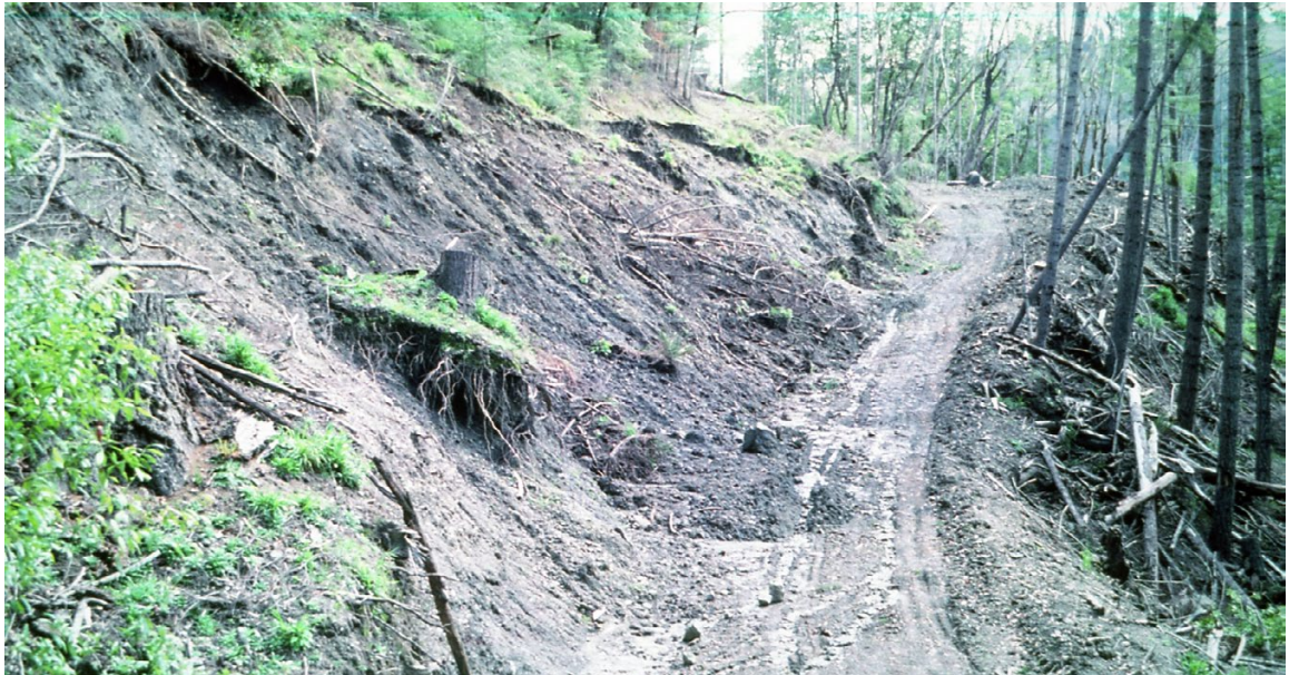
FIGURE 56. This forest road was constructed through wet, unstable soils and subsequently experienced shallow slope failures and rapid erosion rates for a number of years following road building.
