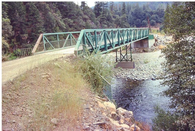
FIGURE 119. It is important that all bridges used to transport vehicles and equipment be properly designed or evaluated by a structural engineer before they are put into use. This long, truss-reinforced bridge was fabricated from two 90-foot long railroad flatcars with a center pier support that can be folded up under the bridge during winter flood flows. The center pier must be put down to haul heavy loads across the bridge.
