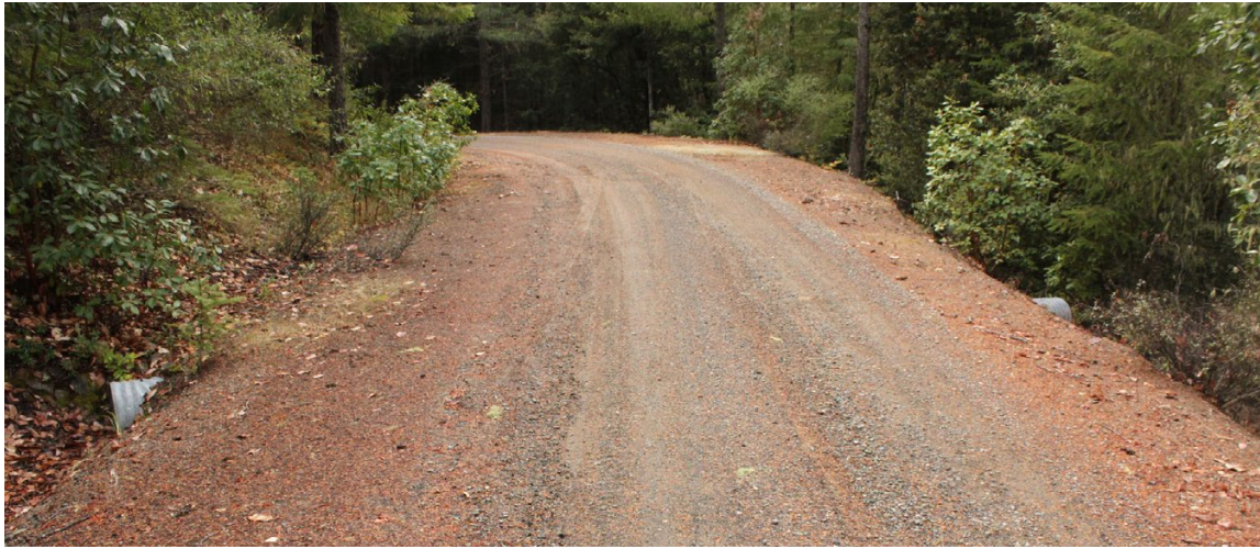
FIGURE 48. The elements of a properly installed ditch relief culvert. The culvert is angled at about 30^\circ to the road alignment to help capture flow and prevent culvert plugging or erosion of the inlet area. It is set at the base of the fill (ideally) or with a grade slightly steeper than the grade of the contributing ditch (but never with a grade less than 2 percent). At a minimum, the grade of the ditch relief culvert should be sufficient to prevent sediment accumulation at the inlet or deposition within the culvert itself (it should be self-cleaning) (USDA-SCS, 1983).
