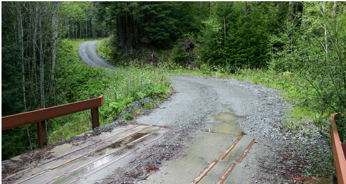
FIGURE 86. Rolling road grade is one method used to effectively drain a road and disconnect road runoff from streams. This road was dipped and then rises to the bridge crossing, ensuring that road runoff is drained off the road and onto the vegetated hillslope prior to reaching the crossing.
