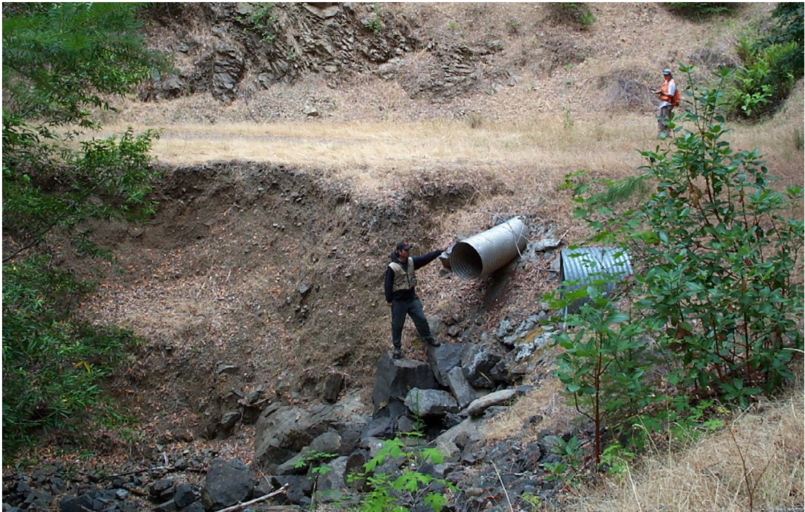
FIGURE 256. Unmaintained, culverted stream crossings, like this one, will eventually plug and either wash out or divert streamflow down the road. Most abandoned roads have drainage structures that are very undersized and often rusted through. Damage from the diversion of even small streams can cause large gullies or debris slides when released on steep, erodible slopes.
