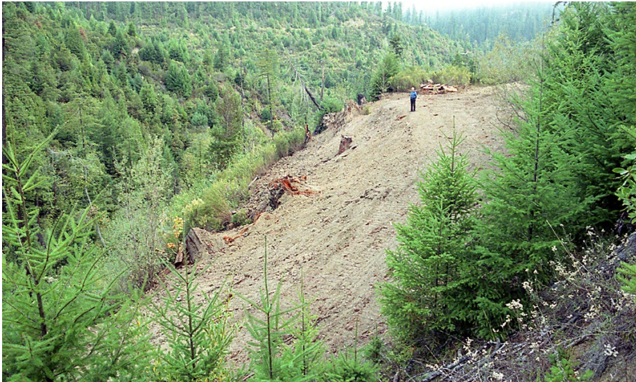
FIGURE 272B. The excavation required a temporary road be built across the middle of the long fill slope to reach all the unstable material. The concave excavation surface mimics the shape of a potential slide plane and thereby assures that most of the unstable fill material has been removed. Spoil materials were pushed up against the inside of the large landing, entirely on a stable, excavated bench. As in Figure 271B this type of out-sloping is called an “Inplace Outslope” (IPOS), where all the excavated materials were stored locally (note person for scale).
