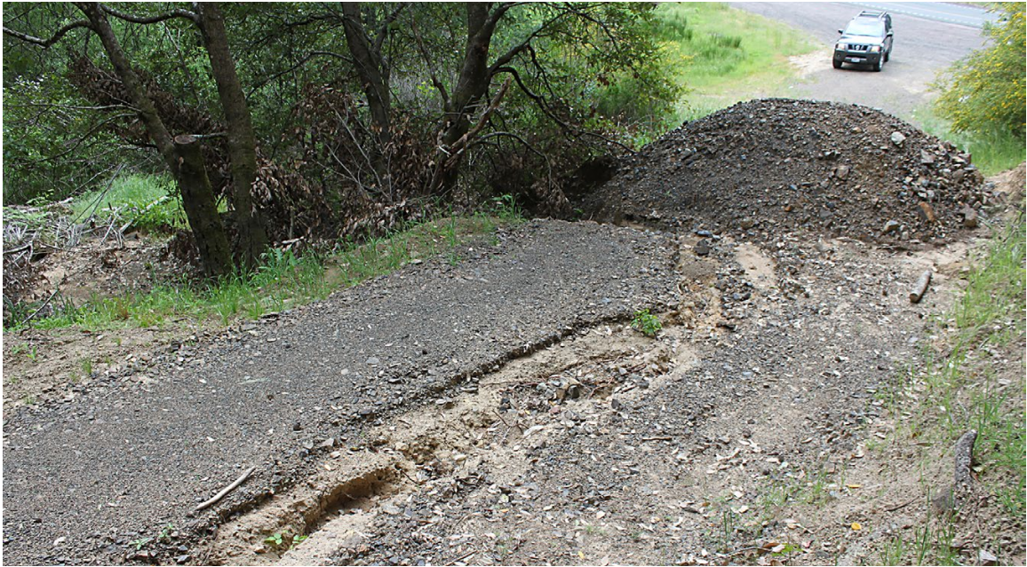
FIGURE 258. Recently constructed barrier blocks access to an unmaintained road, but undrained surface runoff has already gullied the road behind the barrier and now delivers eroded sediment to a stream. Road and storm maintenance cannot be performed when large barriers are constructed. Immovable road barriers should only be installed on roads that have been properly decommissioned.
