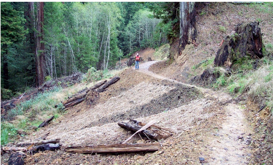
FIGURE 277B. The former road was decommissioned by excavating the sidecast fillslopes and placing the excavated fill against the dry cut banks. The excavated fillslopes were covered with rice straw and woody debris to control erosion while preventing the introduction of exotic grass and weed species. The once-straight road has been converted into a winding trail that follows the original landscape contours. Topographic swales and stream channels have all be excavated and recontoured
