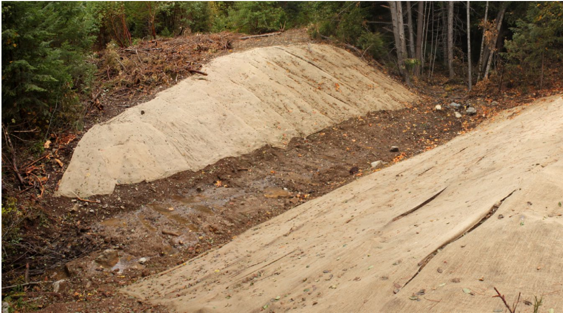
FIGURE 287. Most often, a uniform cover of straw mulch is all that is needed to temporarily control surface erosion on the excavated sideslopes of decommissioned stream crossings until they can naturally revegetate. Wood chips, or native brush and slash, also work well to control surface erosion in some environments. Here, jute netting has been used instead of straw, as a trial treatment. Rolled and tacked erosion control blankets, or jute netting tacked over a layer of straw mulch, can be used on sideslopes that are steeper than about 2:1 (50%). To avoid spreading non-native weed species, many areas can employ rice straw whose seed and weed species are not adapted to growing in most upland environments. Rice straw mulch also has a roughness or “stickiness” that allows it to hold in place on slopes steeper than wheat or grass straw.
