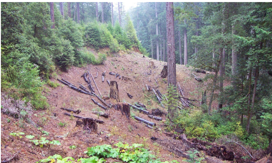
FIGURE 274B. After treatment, remnant stumps that had been buried by road construction and sidecasting were exhumed and gave the excavator operator a good idea where the original ground surface had been located. The outsloping was performed with little or no endhauling, as fill materials from the outside of the road prism were excavated, placed and compacted against the dry cutbank. Most of the cutbank has been buried and the slopes recontoured to their original form. The exposed soil was not seeded with grass, and rice straw was used as a mulch to prevent the introduction of non-native weeds. Litter from the adjacent forest quickly covered the surface.
