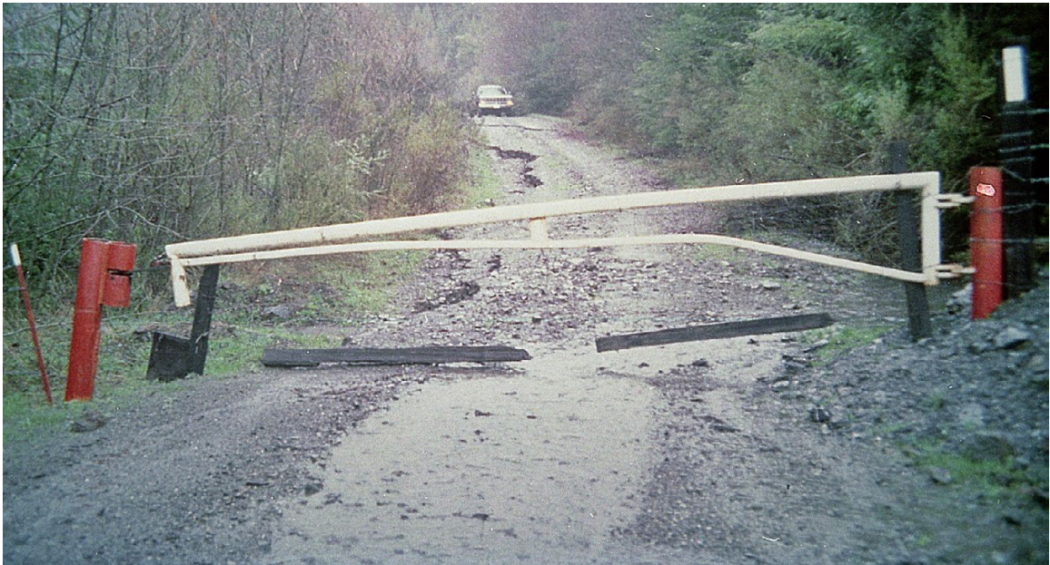
FIGURE 259. Gating a road closes it to unauthorized traffic and may reduce surface erosion, but does nothing to protect the road from major failures. Scarps in the road fill behind this gate signal a slope failure that threatens to deliver sediment to an adjacent fish-bearing stream if it is not treated.
