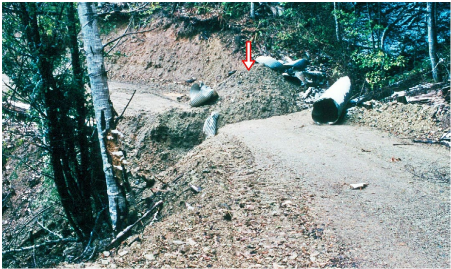
FIGURE 264. Poorly “decommissioned” stream crossing where the culvert was removed by trenching and the excavated spoil was piled next to the trench (see arrow) where it could easily erode into the stream. The entire stream crossing fill will be rapidly eroded and delivered to the stream if correct excavation and decommissioning treatments are not implemented before the next runoff event.
