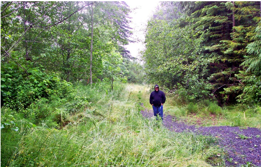
FIGURE 279A. This former (abandoned) forest road crossed relatively gentle topography that had been recently converted to a public use area. The road was to be decommissioned to remove the potential erosion threats, while at the same time opening trail access to the public. Note the conifer tree partially visible in the center background, behind the deciduous alder trees.
