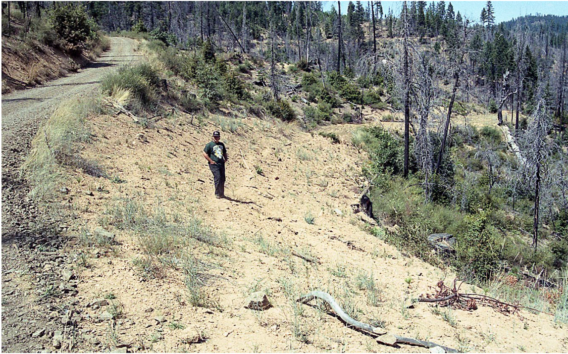
FIGURE 292. Severe outsloping, which prevents vehicle access, should only be used on temporary roads and decommissioned roads where all stream crossings have first been removed, unstable fill slopes have been excavated or stabilized, and road surface drainage is permanently dispersed. To help ensure vehicles do not use the closed road, logs, boulders and brush can be spread over the surface, especially near the beginning of the road, to discourage unwanted traffic. These roads should need no future maintenance, so vehicle access is no longer needed.
