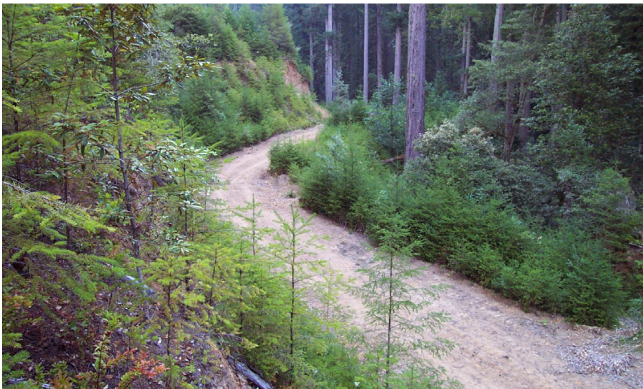
FIGURE 274A. Abandoned forest road that was reopened for decommissioning and erosion prevention treatments. The proposed treatment was to completely restore and recontour the hillslope in this biological reserve and conservation area.
