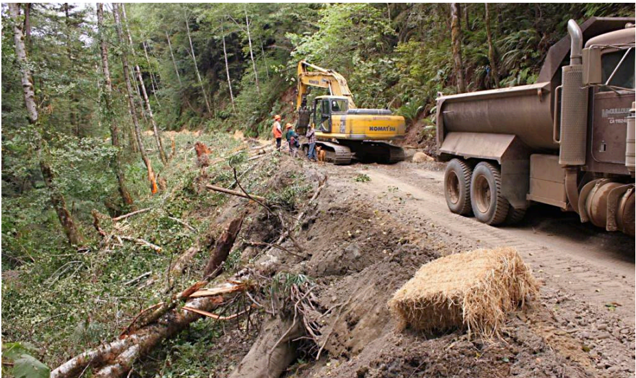
FIGURE 271A. This abandoned, inner gorge road was targeted for permanent closure (decommissioning) because of the steep slopes, unstable road fill and the proximity of a fish bearing stream. Vegetation has been cut from the fill slope and straw bales have already been staged along the road for mulching after the heavy equipment work is complete. Most of the decommissioning involved endhauling spoil about 1000 feet down the road to a broad, low gradient area located far from the stream.
