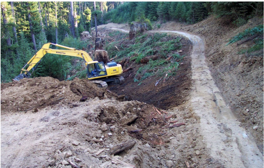
FIGURE 276. This road-to-trail conversion (decommissioning) was undertaken when the forested area, once commercial timberlands, was acquired and converted to a biological preserve. Part of the ecological mandate was to decommission former logging roads to reduce erosion rates to protect streams and fish habitat, while still preserving hiking access to many of the biologically unique areas. Here an excavator is recontouring a former logging road while constructing a new trail near the top of the old cut slope. The surface of the recontoured slope has been mulched with limbs and woody debris. All stream crossings and unstable road fills have been excavated along the old road alignment.
