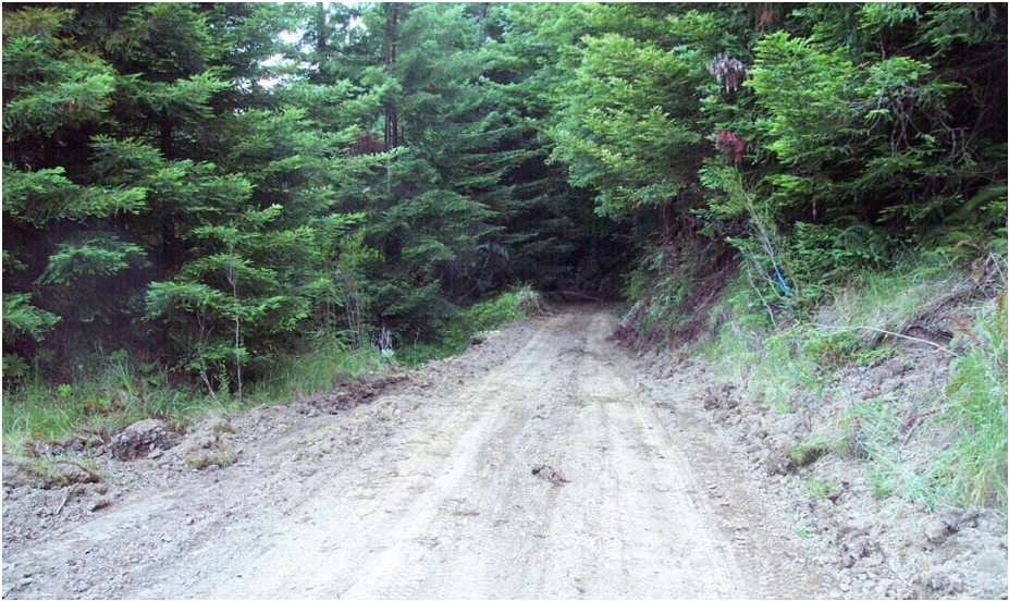
FIGURE 269B. This low standard forest road was scheduled for decommissioning because of slope stability and erosion problems along its alignment. Prior to road grading, inventory crews had identified cracks and small scarps along 50 feet of the road bench and outer fill. If it failed, the debris slide would deliver sediment to a stream just downslope.
