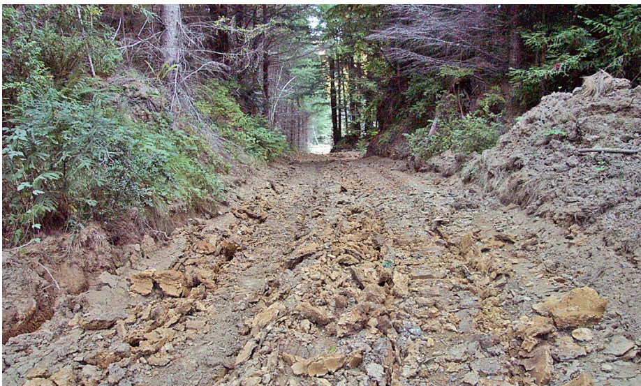
FIGURE 284B. A road after ripping and decompaction.
