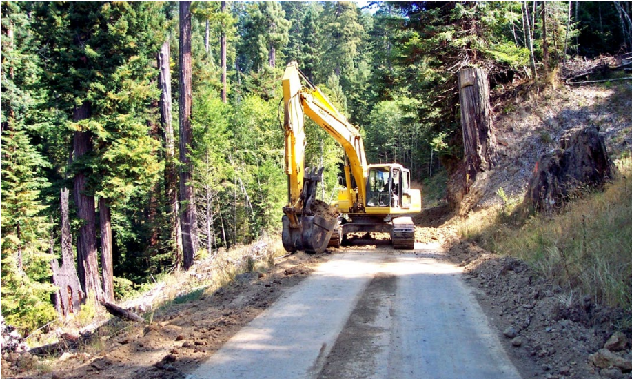
FIGURE 277A. Former private forest road, now in a U.S. BLM Biological Reserve, has been scheduled for out-sloping and conversion to a trail. The purpose of the decommissioning project was to recontour the old logging road and convert the route to hiking access for visitors and researchers. Note the stump in the right foreground.
