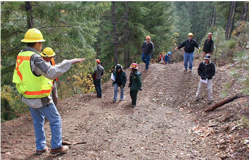
FIGURE 281. Between treated stream crossings and fill slope excavations, decommissioned roads should have permanent road drainage treatments, including road decompaction (ripping or subsoiling) and constructed cross road drains. Cross road drains are permanent road drainage features, like waterbars but much more substantial so they will function indefinitely and will not be broken down by rainfall, runoff or any kind of unwanted recreational traffic (usually bicycles or motorcycles). Like waterbars, they are usually excavated into the firm roadbed, mounded on the downhill side and spaced closely enough to prevent significant erosion on the roadbed or below the point of discharge.
