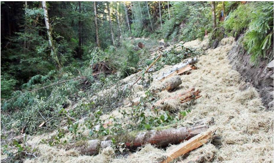
FIGURE 271B. After decommissioning, all the potentially unstable fill material has been excavated and endhauled off-site. Some excavated material has been placed along dry portions of the cut-bank, but seeps and springs have been left uncovered to freely drain down the slope. The excavated fill slope and road bench has been covered with alder trees that were growing on the slope, and the remaining bare soil areas were seeded and mulched with straw. The threat to the stream at the base of the slope has been eliminated.
