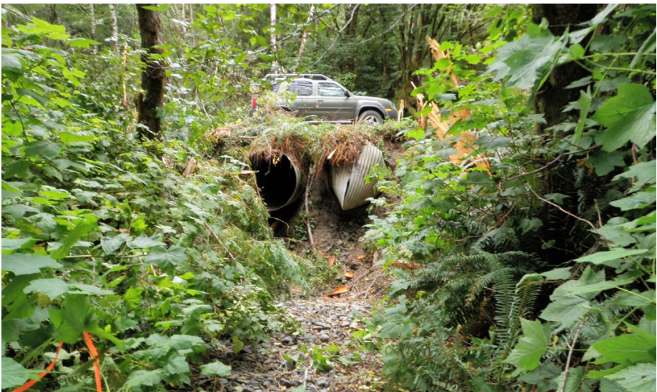
FIGURE 267A. Dual, undersized, elevated culverts at this small stream crossing have been a barrier to fish passage since the road was built decades ago. The outlet of the culvert on the right has been crushed closed, probably by heavy equipment performing maintenance work. Road and stream crossing decommissioning was used to permanently reopen the channel to fish passage.
