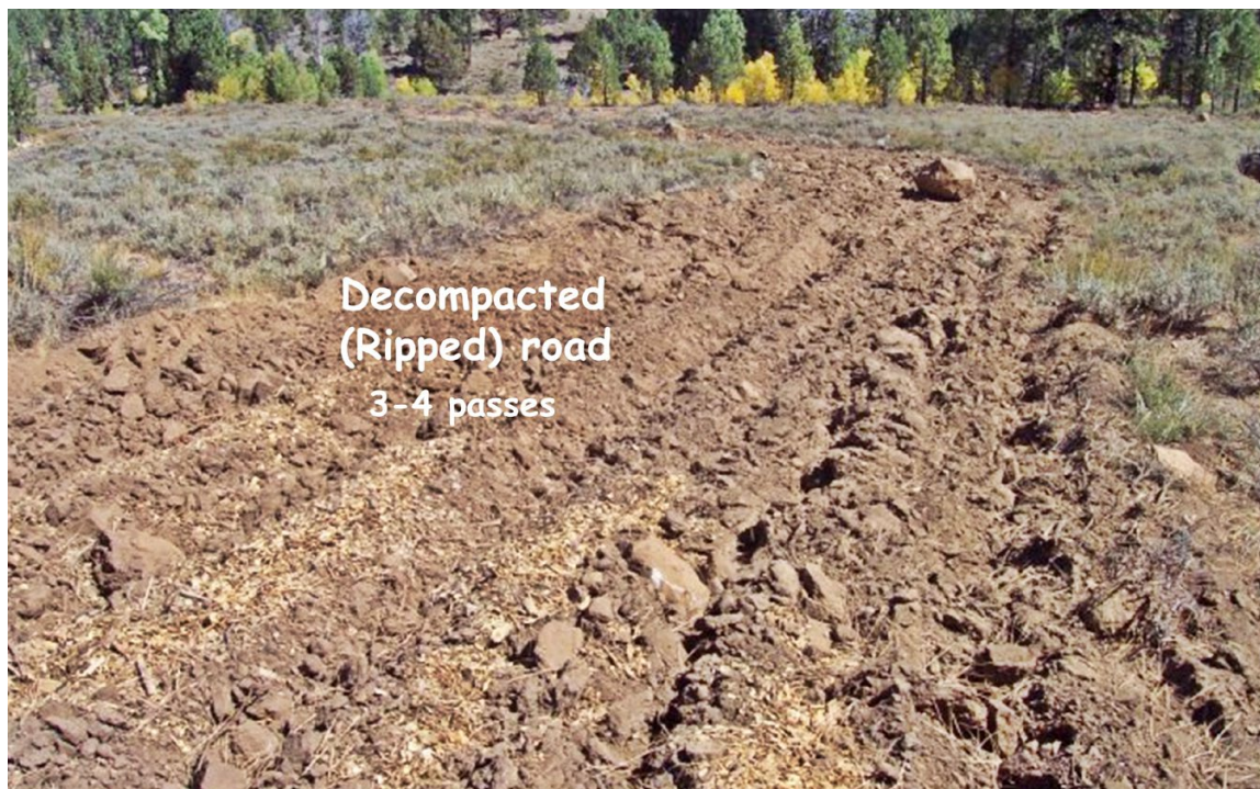
FIGURE 286. On gentle terrain, ripping (soil decompaction) maybe the only treatment that is needed to decommission a road, eliminate unwanted traffic, reduce runoff and return it to native vegetation.
