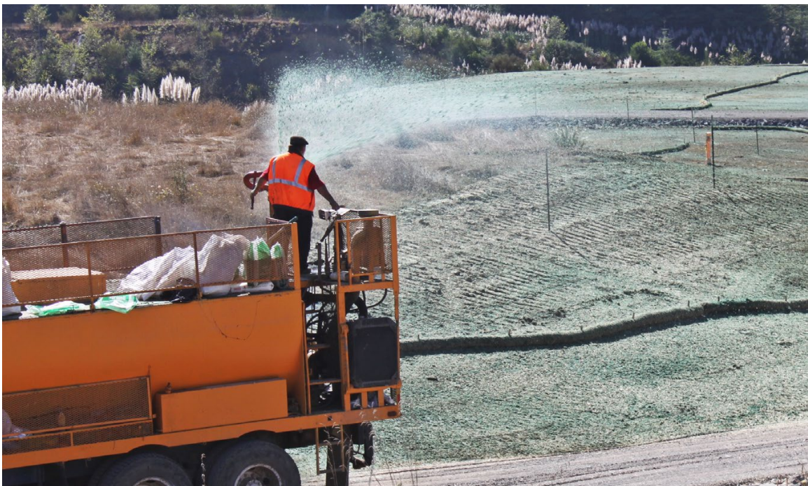
FIGURE 288. Hydroseeding (spraying a slurry of water, mulch, seed and fertilizer) on bare soil areas can be an effective erosion control and revegetation treatment for large disturbed areas, or for bare soil areas along open roads. It is most useful for treating spoil disposal sites, after they have been graded and smoothed, and for treatments along newly upgraded roads where the truck or trailer can have easy access. Hydroseeding decommissioned roads is more difficult because access is cut off as the treatments progress. Rather, hand seeding and mulching is usually the preferred treatment.
