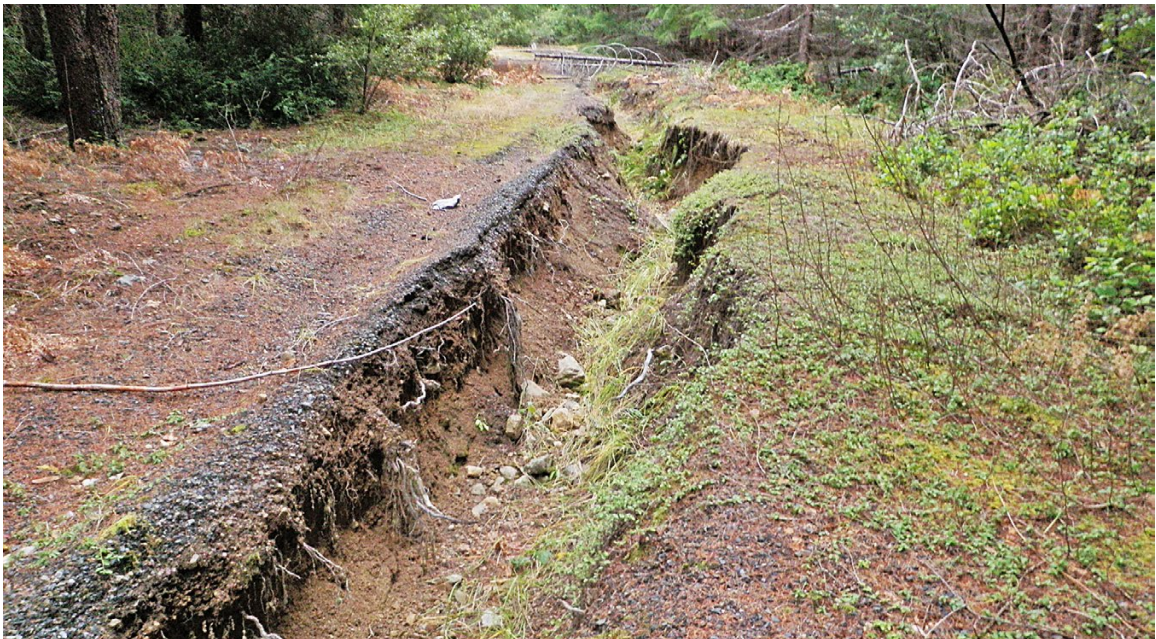
FIGURE 255. Gully formed by culvert plugging and stream diversion on an old, unmaintained forest road. The degree of threat posed by old roads depends on the terrain the road crosses. Typically, the most serious threats occur where roads cross stream channels and steep, wet and/or unstable hillslopes.
