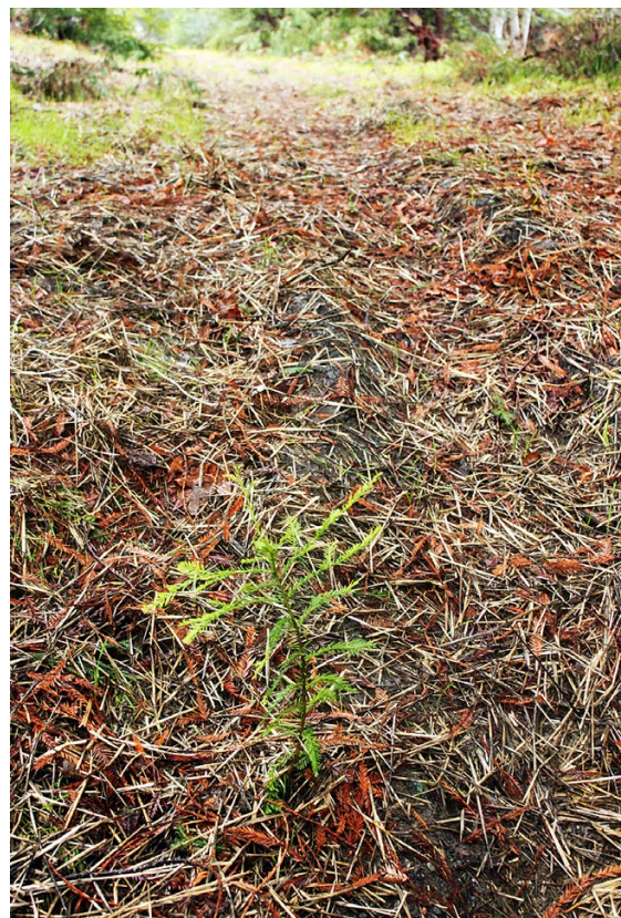
FIGURE 289. Tree planting (or planting woody species suitable for the specific environment of the road) is the final long term treatment for the decommissioned roadbed and for the riparian sideslopes where stream crossings have been excavated and restored for the long term. This planted redwood tree, and those conifers and hardwoods that naturally seed themselves onto the former roadbed, will eventually cover the alignment and provide for long term site stability.
