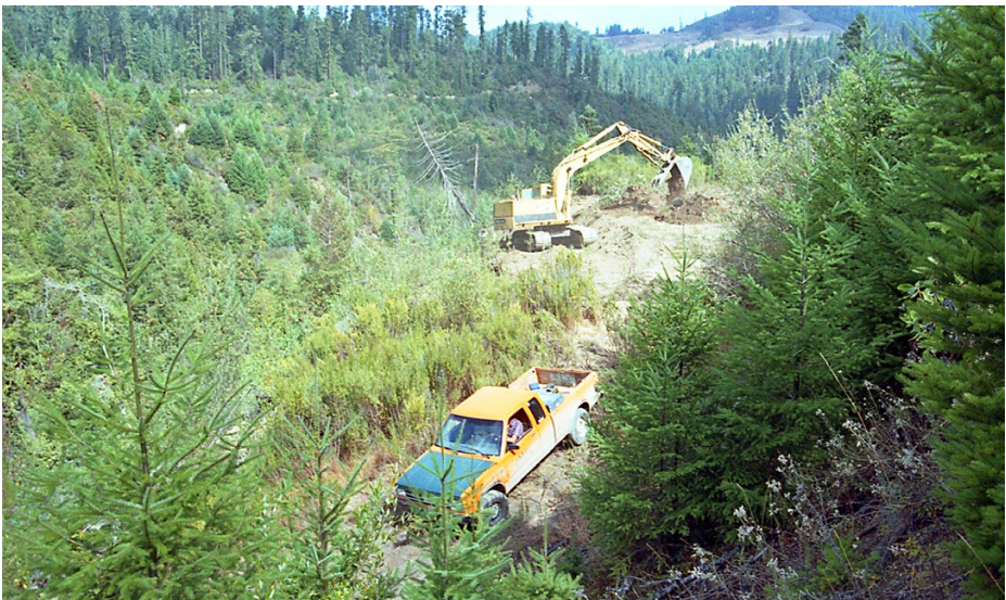
FIGURE 272A. Log landing on a forest spur road had developed large cracks and scarps around its outside perimeter where soil and wood waste had been sidecast onto steep slopes above a fish bearing stream. The fresh scarps had developed over several years and were identified by an inventory crew surveying for erosion problems in the watershed. An excavator is beginning the fill slope excavation and spoil material was pushed against the inside of the landing by a bulldozer (not visible).
