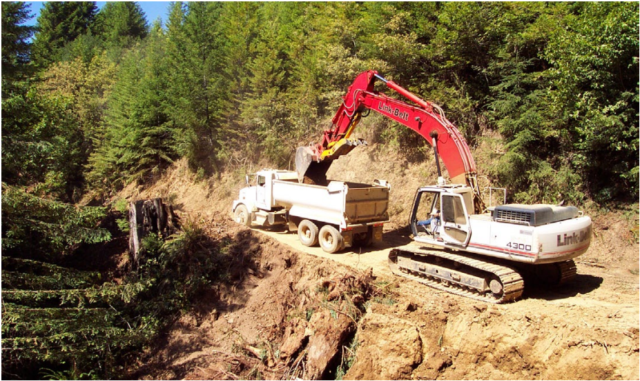
FIGURE 269A. Hydraulic excavator loading a 10-yd 3 dump truck with fill material removed from an unstable road fill slope. The road decommissioning process whereby excavated spoil is endhauled off site, rather than placed against the cutbank, is call “Export Out-slope” (EOS). EOS is used where unstable fill material must be excavated, but the cutbank is unstable or wet and cannot be buried. Spoil is endhauled to the nearest stable disposal site.
