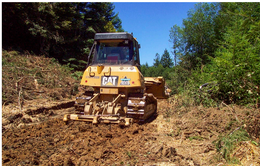
FIGURE 283. Small bulldozer with hydraulically operated rippers (three 30 inch long steel chisels) is decompacting a seasonal road as a part of road decommissioning. Road ripping should be a standard decommissioning practice. All decommissioned roads should be ripped to decompact the road bench, improve and speed revegetation and reduce surface runoff. If the road is to be outsloped, and spoil is placed on the former roadbed, the compacted road bench should first be ripped to a depth of 18 to 24 inches, or greater. If it isn't ripped, infiltrating water will pond on the compacted surface and may cause soil saturation or contribute to slope failure.
