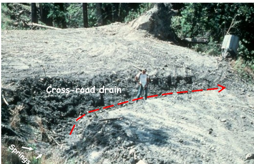
FIGURE 282. Deep cross road drains are constructed everywhere there is a spring or seep on the former road cutbank. This helps drain the road and the hillslope as uniformly and frequently as possible. Except for very short sections next to a cross road drain, inside ditches should not be retained.
