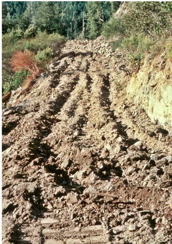
FIGURE 290. Deep, thorough ripping is a good treatment to largely eliminate surface runoff and “hydrologically disconnect” a former road from nearby stream channels.
