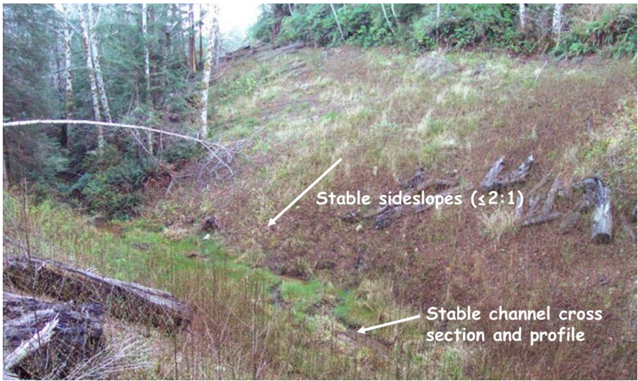
FIGURE 265. Properly decommissioned stream crossing, with 2:1 (stable) sideslopes, adequate channel width for flood flows, and a uniform channel grade (no humps of unexcavated fill) extending between the natural channel above and below the crossing. Because the slopes were dry, excavated spoil material was used to outslope the adjacent road approaches. The sideslopes were seeded with grass and straw mulched to minimize erosion following decommissioning.
