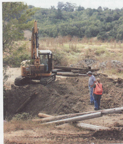
Above: SPAWN, with PWA, replaced an old culvert at Flanders Ranch and regraded the adjacent road to decrease sediment and run-off flowing into the seasonal creek.
